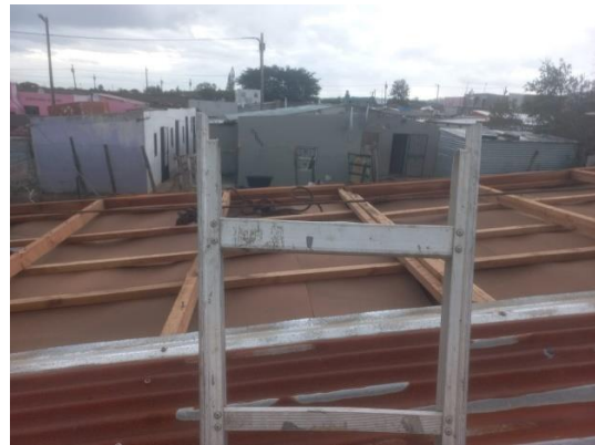
Missing Roof Sheets
